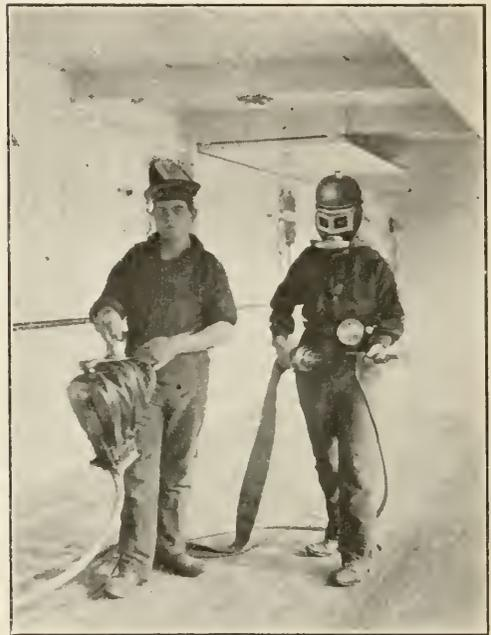
The Fire Helmet with its Air Supply enables the Crew to Enter a Burning Hold and Fight Fire
